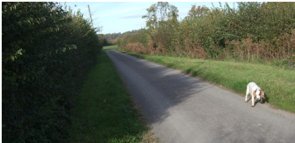
Continuation of road u/c 7008 north
